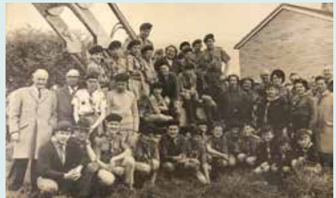
On the Scout hut site before the building went up in 1970
